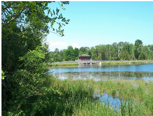
Photograph of the historic power generating dam.
